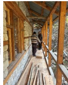
Fig 13: Corner junction of the built mass. Source: (Pandey, 2024)/ exposed kathkuni walls during construction at the homestay. Source: author
