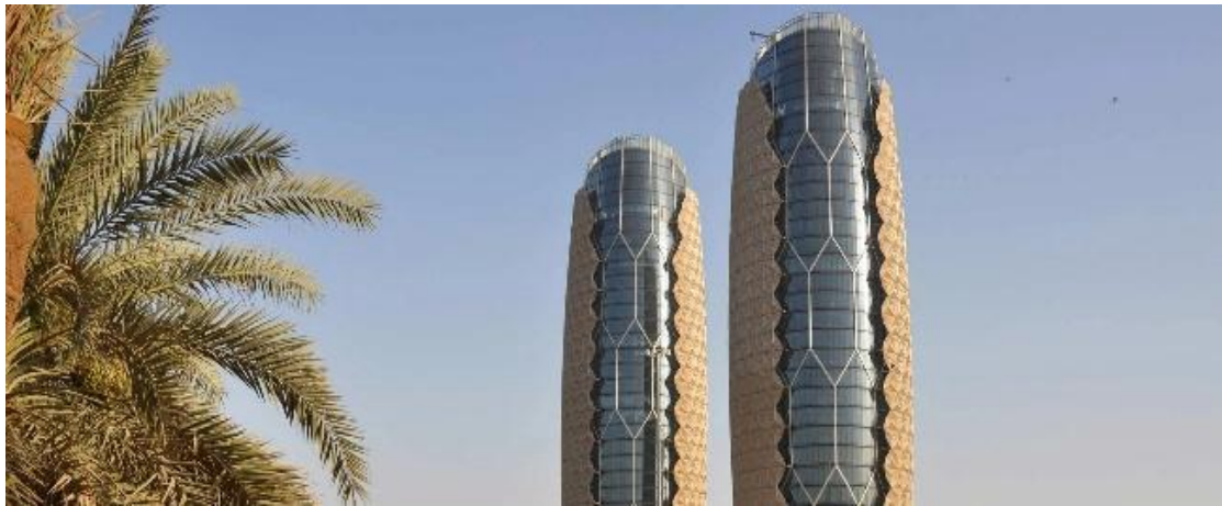
Fig. 1: Al Bahr Towers, Abu Dhabi, UAE
