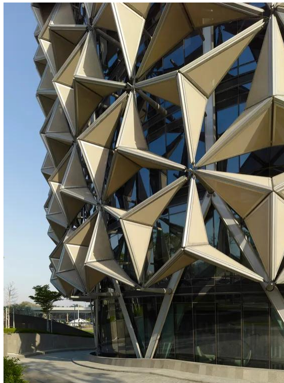
Fig. 2: A detail of the Mashrabiya - Al Bahr Towers, Abu Dhabi, UAE
