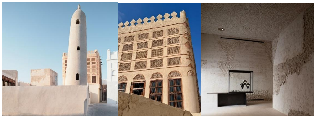
Fig 4: The ensemble (the house, the majlis, the mosque) built by Ahmed bin Jasim Siyadi Source: Anne Holtrop
