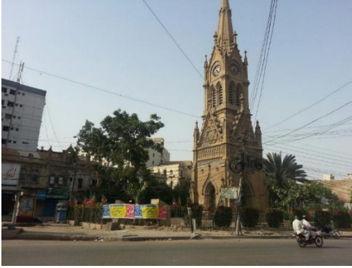
Fig. 9: Electrical Lines around the tower.
