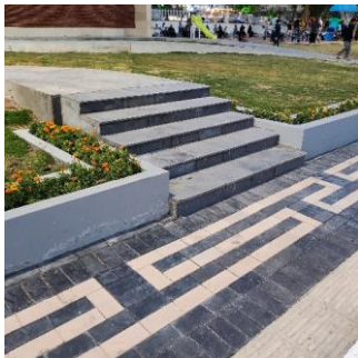
Fig. 15: There is no tactile surface to warning visually disabled people about the step, or a ramp to make connections between the different levels.
