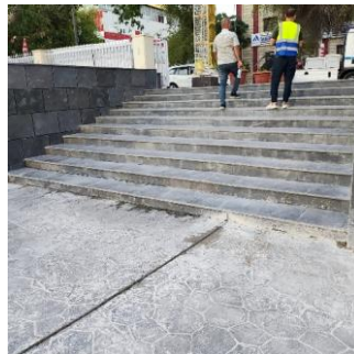
Fig. 15: There is no tactile surface to warning visually disabled people about the step, or a ramp to make connections between the different levels.
