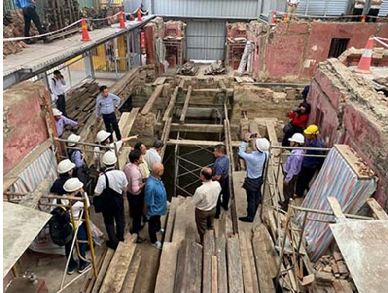
Fig. 3: The Chùa Cầu being officially dismantled and completely taken apart in December 2022, for the most fundamental restoration in its history, – Source: Thái Bá Dũng
