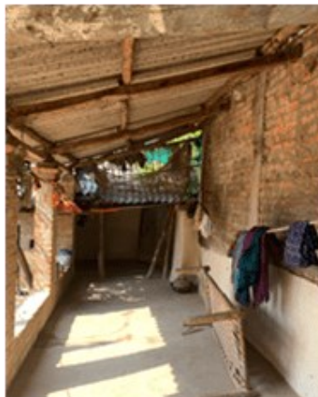
Fig. 11: Change of the wall materials, use of brick piers and asbestos roofs
