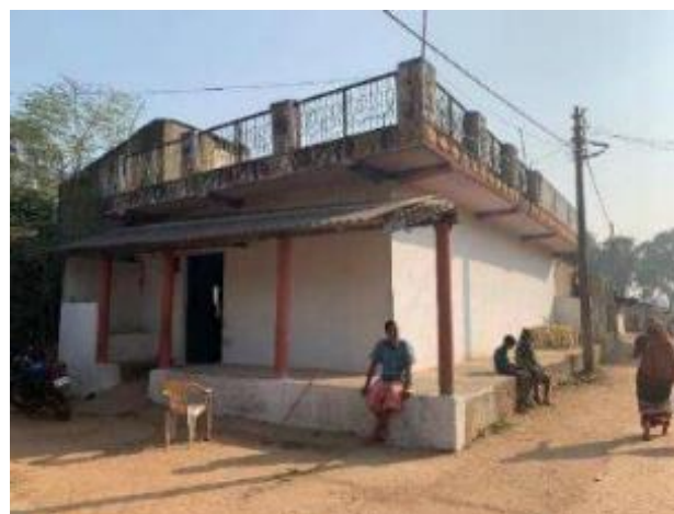
Fig. 13: Addition of a new structure
