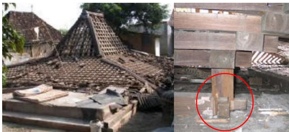
Fig. 3: Joglo which completely collapsed due to the 2006 earthquake; the four main pillars ( saka guru ) in the core structure ( rong-rongan ) were broken.
